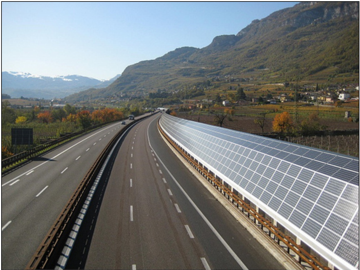
Figure 8 An example of multifunctional integrated solution where photovoltaic cells are integrated into noise barriers.
